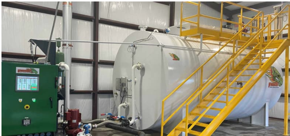
Figure 5-1: Example FOG Separation System Installation
