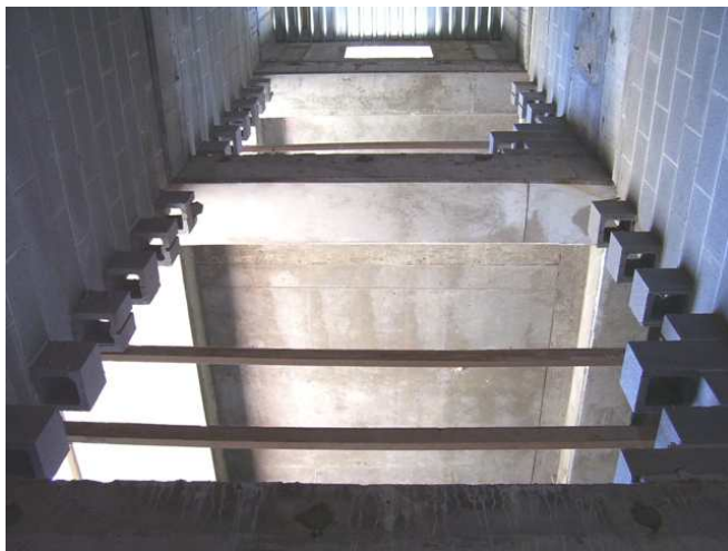
Front wall open before installation of equipment, block wall construction
