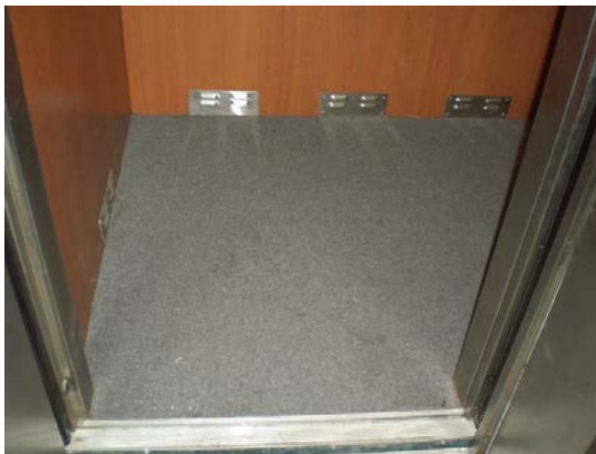
Finished cab flooring
