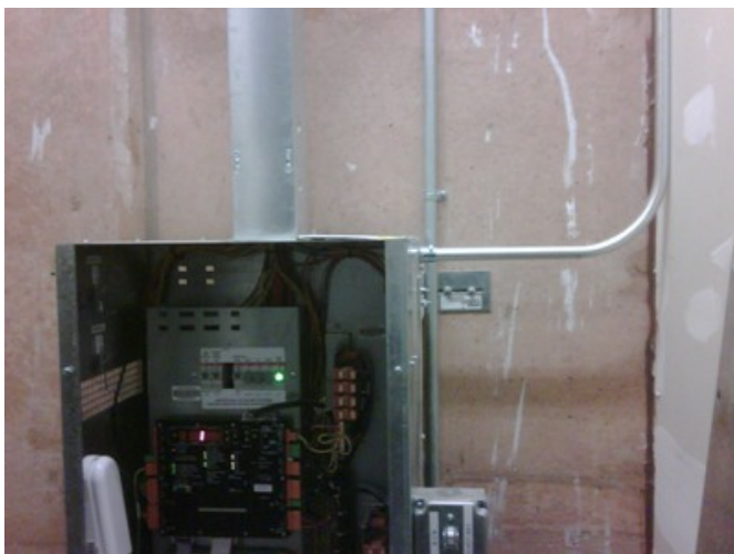
Phone line piping to controller
