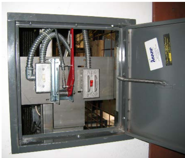
Manual brake release access panel
