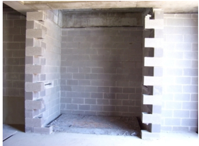
Front wall open before installation of equipment: top landing, intermediate landing and bottom landing
