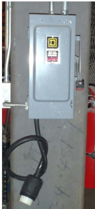
Temporary power for Tirak hoist
