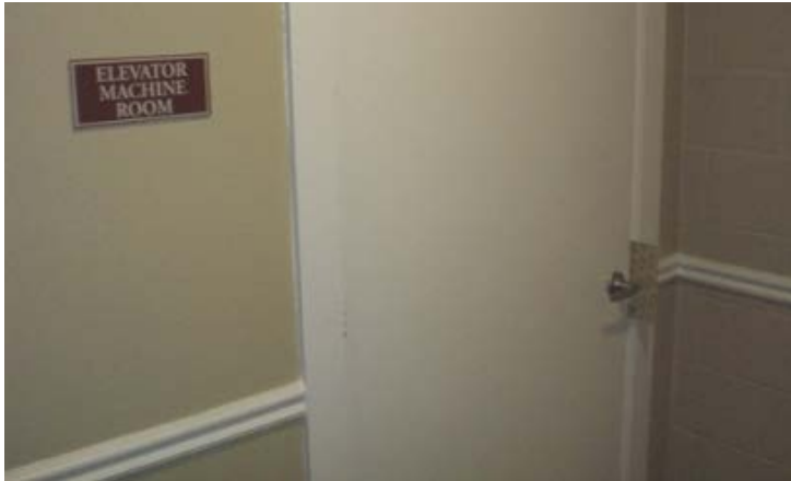
Self-closing, self-locking machine room door
