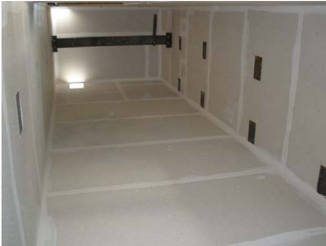
Steel plate attachments in hoistway
