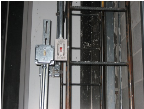
Pit ladder, light switch, stop switch
