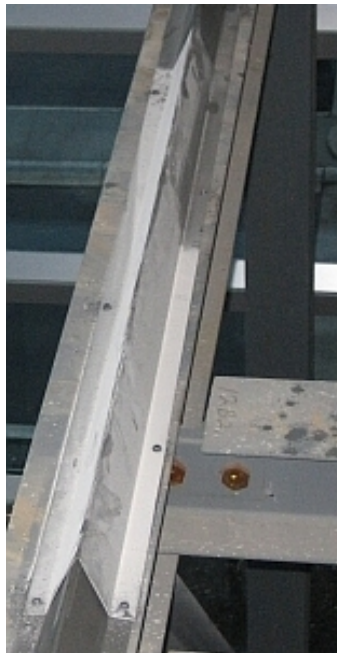
Beveled ledge in hoistway
