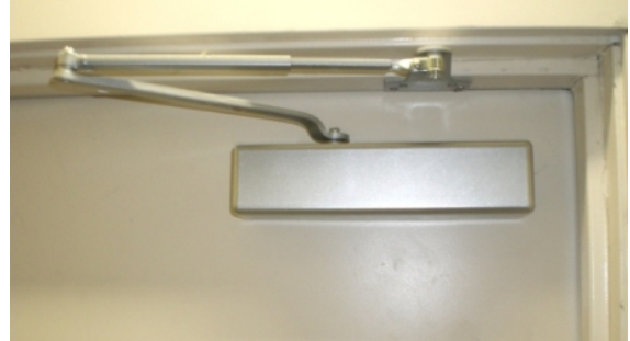
Closer on machine room door
