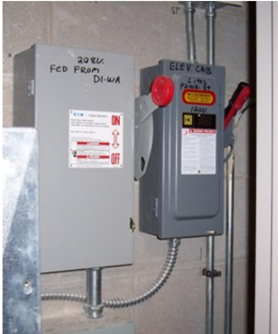
Three-phase disconnects shown on left; car lighting disconnects shown on right
