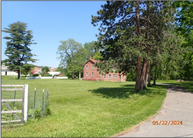
Remaining building on larger parcel
