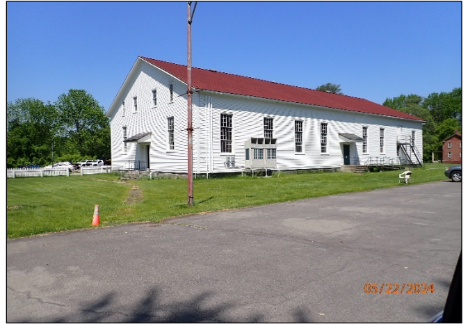
Remaining building on larger parcel
