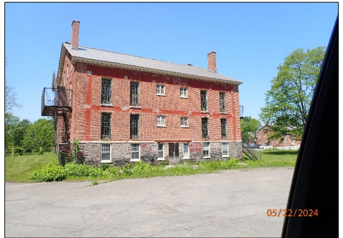
Remaining building on larger parcel
