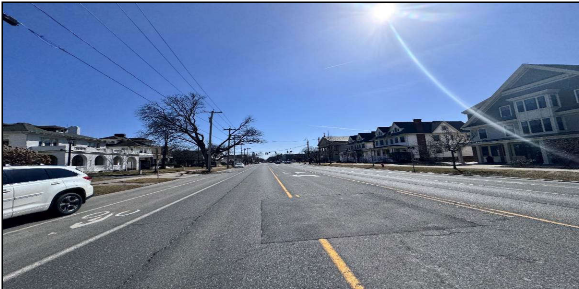
Facing east on Madison Avenue
