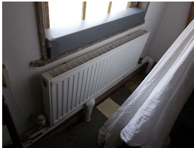
Typical steel hot water radiator with thermostatic valve (at left)
