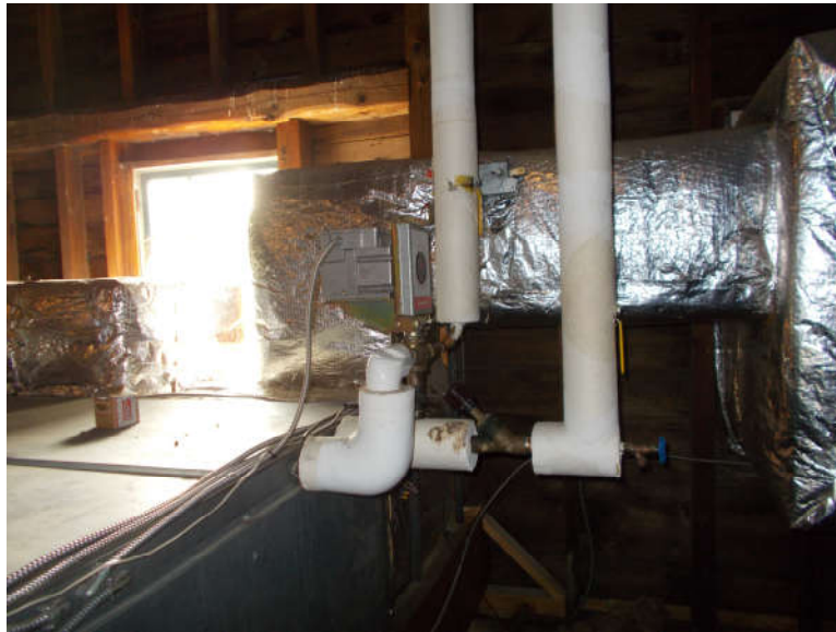
Hot water piping and motorized control valve at air handler
