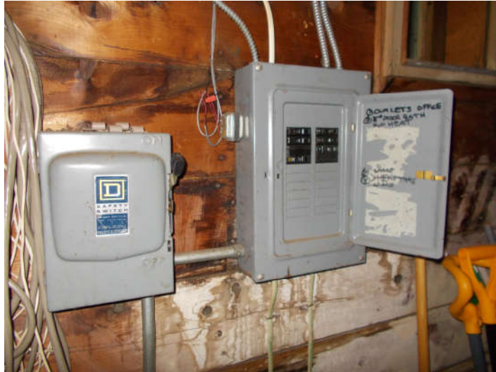
Photo 4 – Attic panel and disconnect switch
