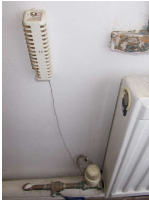
Remote temperature sensor installed on exterior wall.
