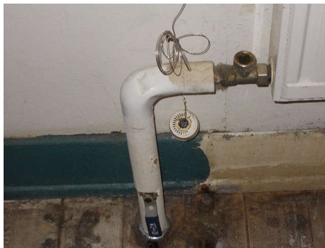
Broken actuator at thermostatic radiator valve
