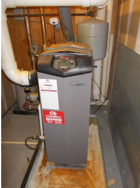
Gas-fired condensing boiler on 3 rd floor
