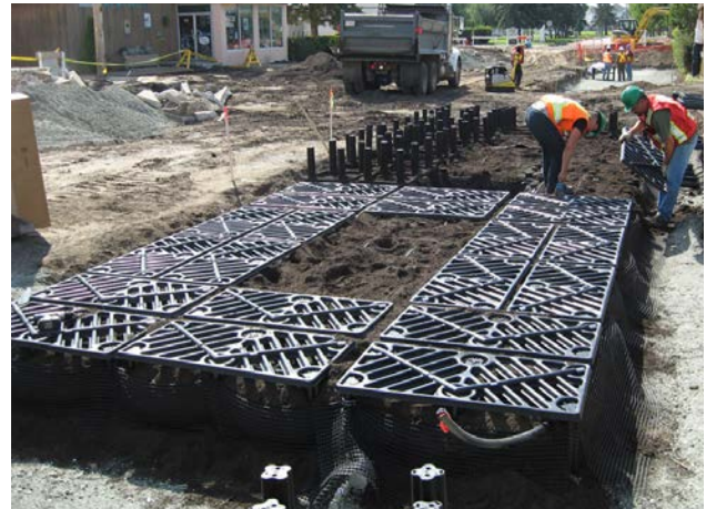
▲ Deeproot Silva Cells are one example of a modular suspended pavement systems that has been used successfully in cities around the world. Image credit: Deeproot
