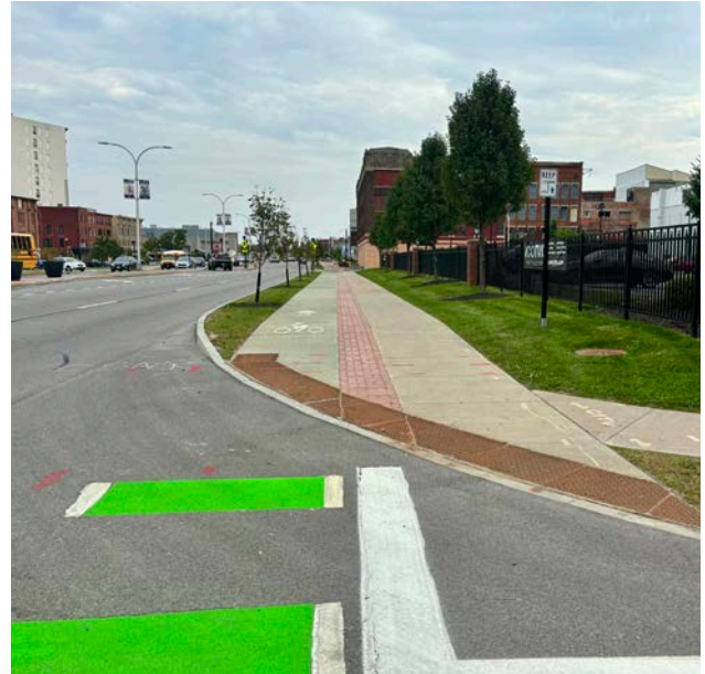
▲ One-way separated bike lane adjacent to sidewalk in Utica, NY.
