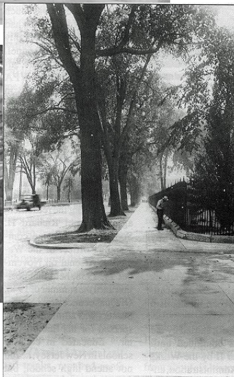
NEW FENCE — New sidewalks and fencing along B were completed under WPA in 1936
