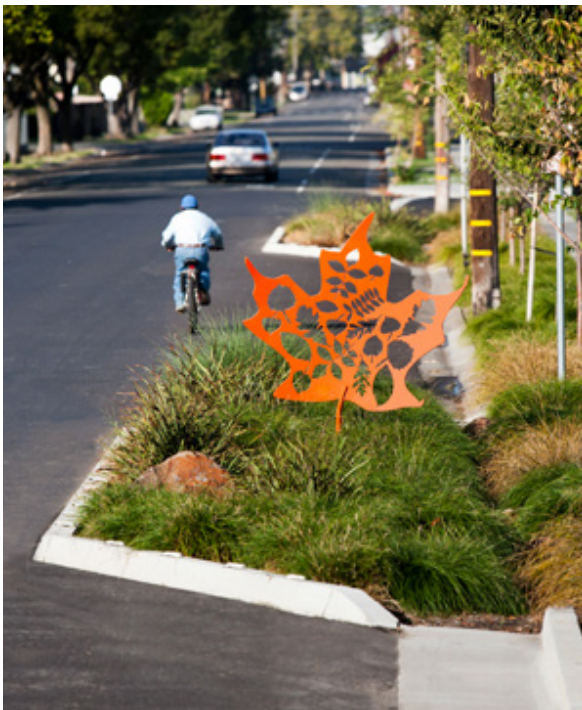
▲ Individual on-street parking spaces can be intermittently replaced with a bioretention island to ensure trees and green infrastructure can still be integrated into the corridor.
