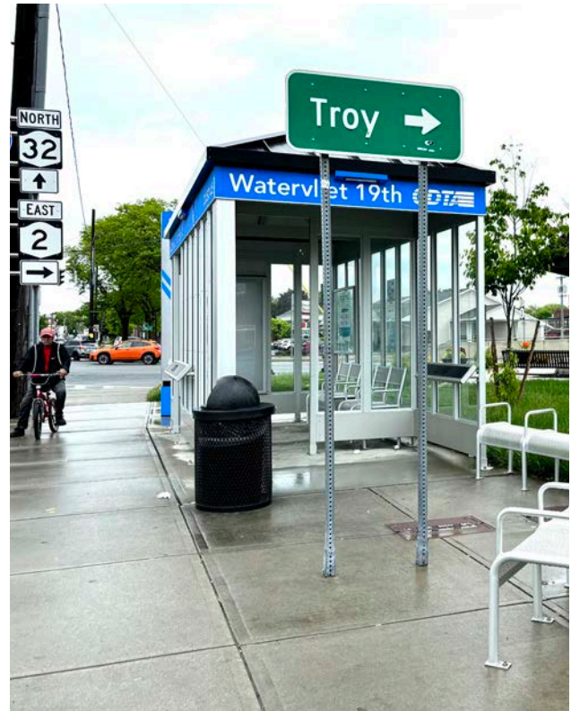
▲ Northbound BRT station at on 2nd Avenue at 19th Street
