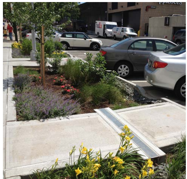
▲ A series of bioswales connected via trench drains in Queens, NY, capture and filter stormwater from sidewalks and the adjacent on-street parking. Image Credit: Chris Hamby / flickr
