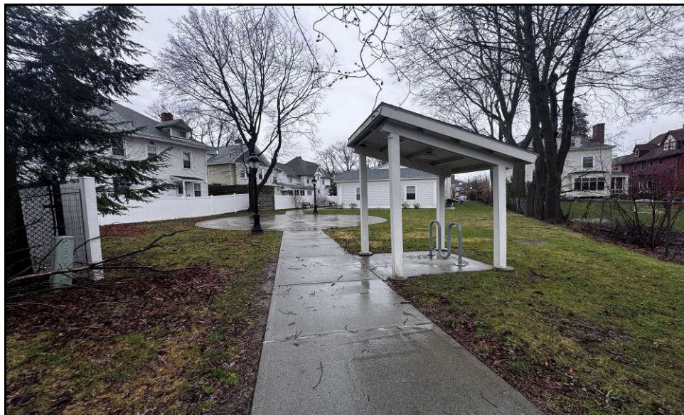
Rear Site Improvements
